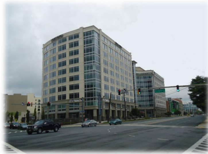
Figure 16: Exterior View from Across Rockville Pike Intersection – by JMV
