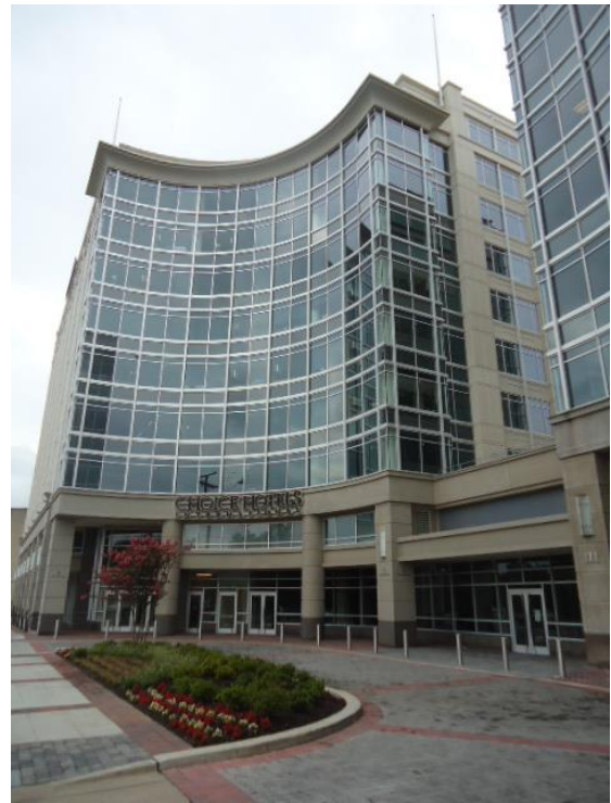
Figure 24: North East Curtain Wall – by JMV
