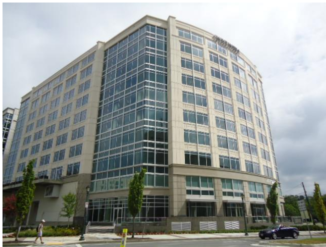
Figure 26: South West Corner – by JMV
